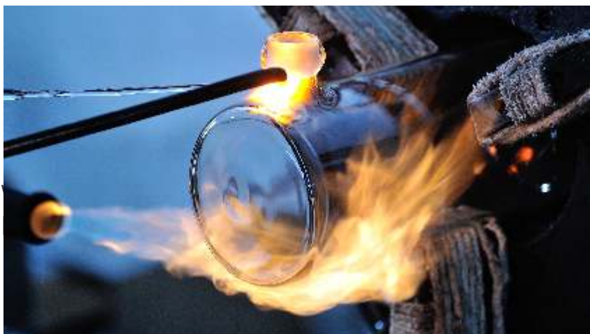
Nozzle fusing in Pipe section
